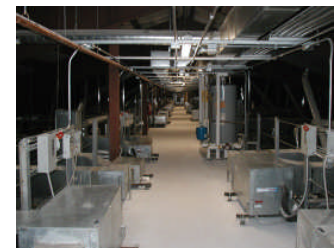
MEZZANINE ABOVE CORRIDOR
