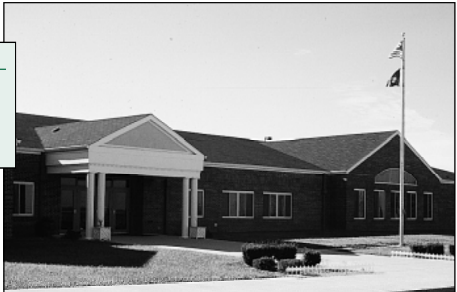
Paint Lick Elementary, heated and cooled by a 123-ton WaterFurnace system, holds the prestige of being the first geothermal school installation in Kentucky.
