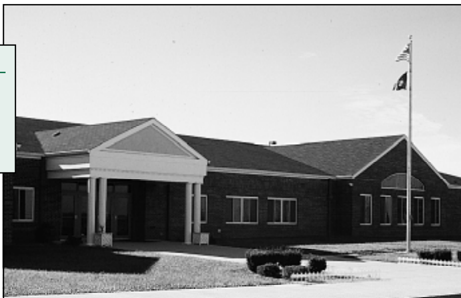
Paint Lick Elementary, heated and cooled by a 123-ton WaterFurnace system, holds the prestige of being the first geothermal school installation in Kentucky.
