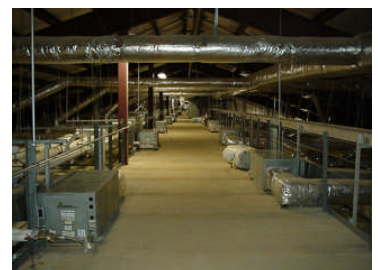
MEZZANINE ABOVE CORRIDOR
